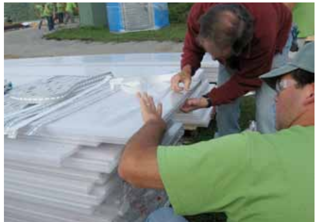
Apply aluminum tape to the ridge edge of each panel and batten.
