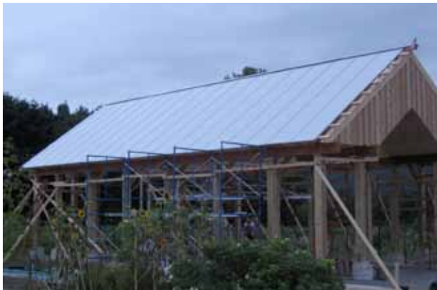
Continue installation across the roof.
